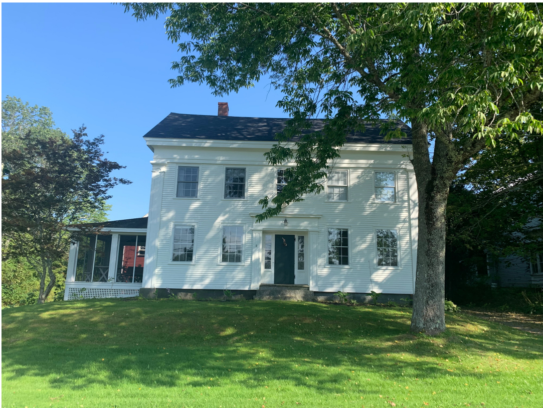
Pictured above: A property within the Sheepscot Village historic district, with a more contemporary screen porch addition.
