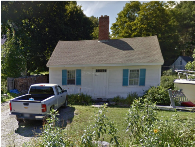
The house pictured above, in the Damariscotta Mills neighborhood, is an example of vernacular construction in Maine from the 1700s.
