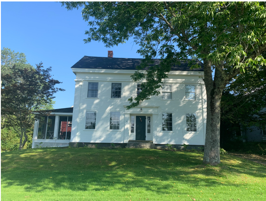
Pictured at left: The enframement of the front door on this Greek Revival home in Sheepscot Village is a character-defining feature of Greek Revival architecture and would not be allowed to be removed under this Standard.
