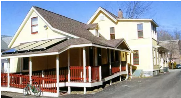
Pictured at left: A property in a Vermont community where solar collectors are installed on a rear roof slope on a newer addition, minimizing impact to the original, historic portion of the building. This would meet the Ordinance standards. Photo c/o U.S. Secretary of the Interior Technical Preservation Services.
