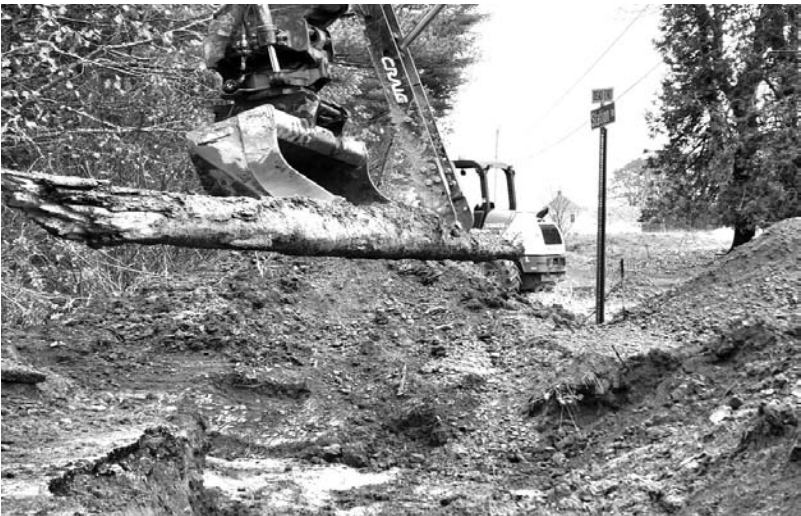
A piece of the log drainage system under the Station & Island Rd. intersection.
