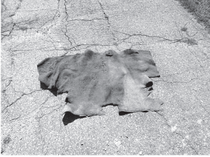
Figure 2A carpet that was found on Academy Hill, used as a patch on one of the old drainage lines. At some point there was a repair made and a rug was used to bridge the hole. This carpet was all that was preventing the road from collapsing
