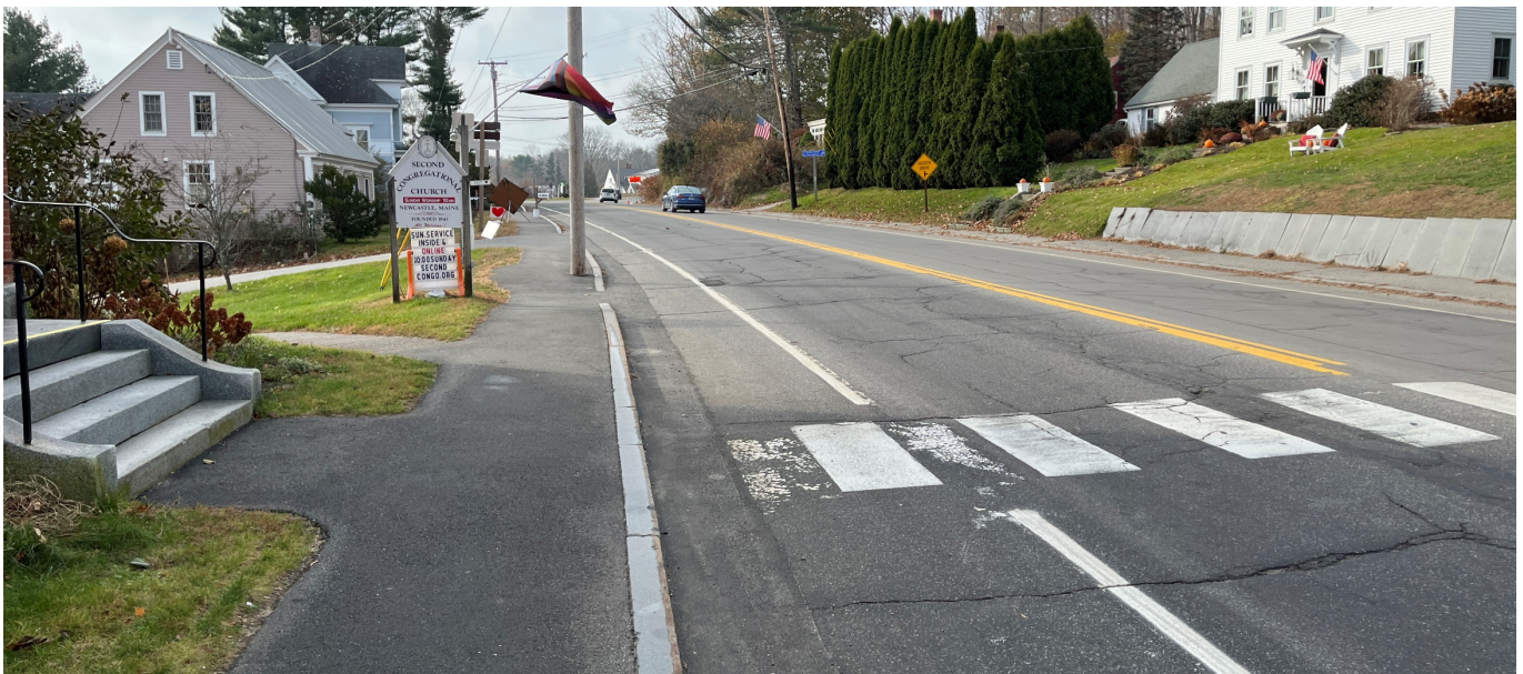
Main Street looking south toward the River Road intersection. Note the crosswalk without ADA accessibility on sidewalk.
