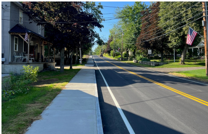
Front Street neighborhood after improvements.
