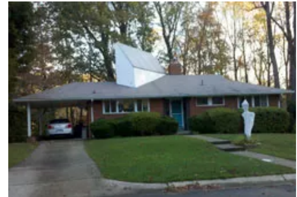
Pictured above: A property in another community where solar collectors are popping up from the roof, negatively impacting the character of this mid-twentieth century house. This would not meet the Ordinance standards. Photo c/o U.S. Secretary of the Interior Technical Preservation Services.
