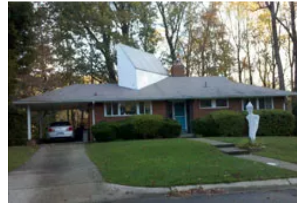
Pictured above: A property in another community where solar collectors are popping up from the roof, negatively impacting the character of this mid-twentieth century house. This would not meet the Ordinance standards. Photo c/o U.S. Secretary of the Interior Technical Preservation Services.
