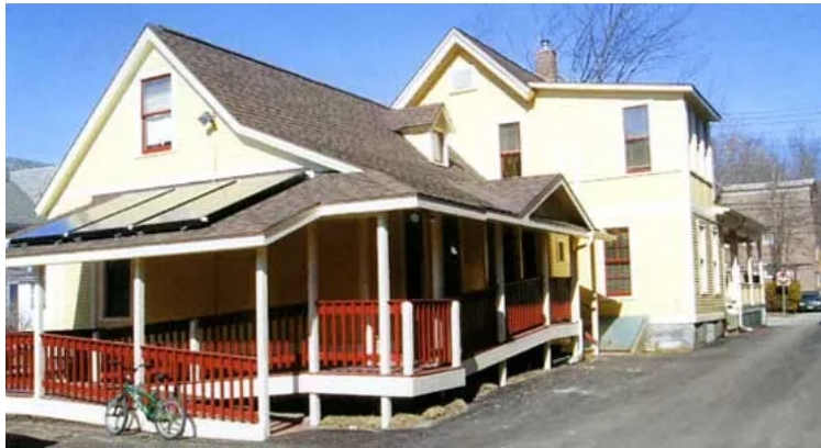
Pictured above: A property in a Vermont community where solar collectors are installed on a rear roof slope on a newer addition, minimizing impact to the original, historic portion of the building. This would meet the Ordinance standards. Photo c/o U.S. Secretary of the Interior Technical Preservation Services.
