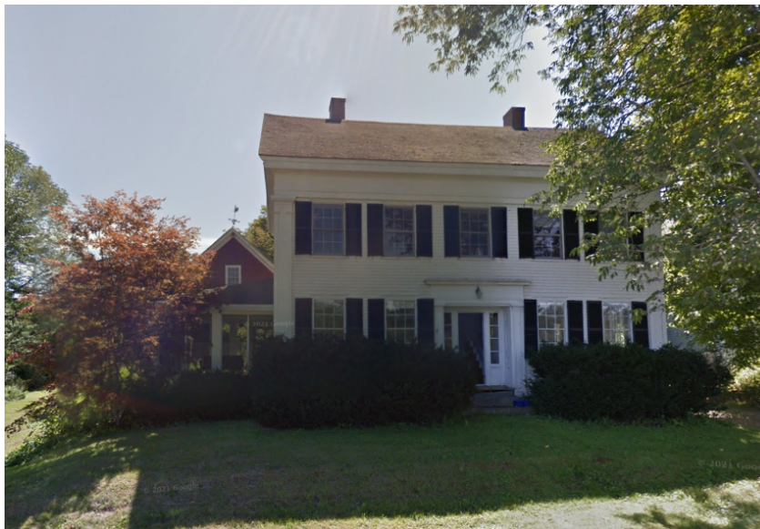
Pictured at left: The enframement of the front door on this Greek Revival home in Sheepscot Village is a character-defining feature of Greek Revival architecture and would not be allowed to be removed under this Standard.
