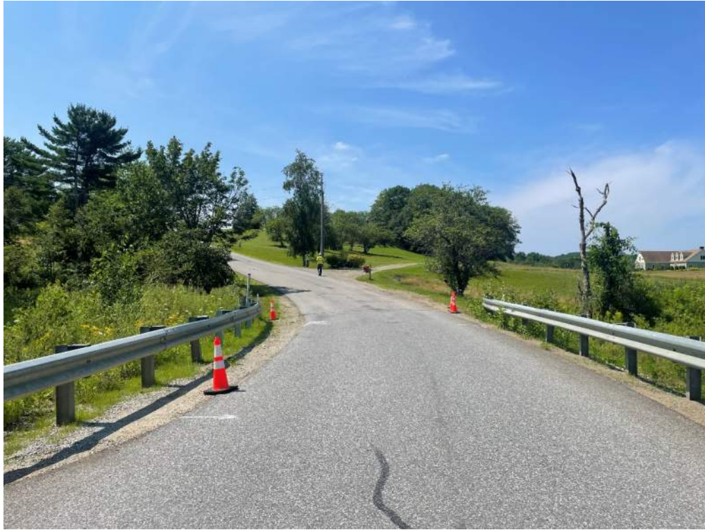
Photo 3: View South along Lynch Rd (Left Approach)
