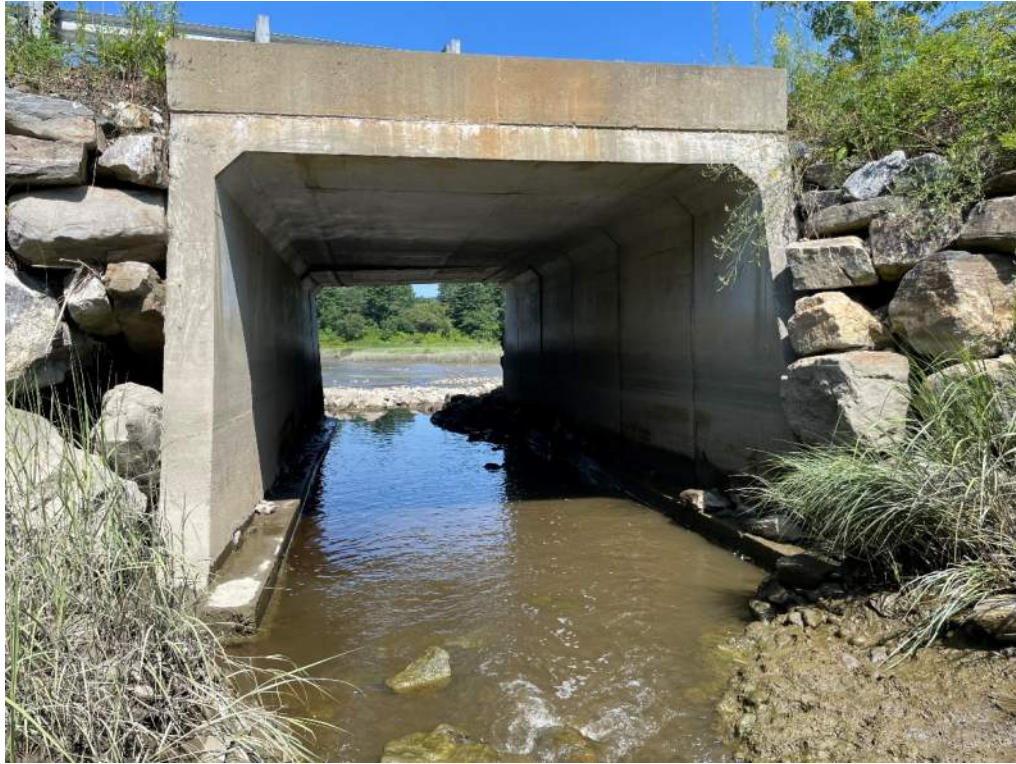
Photo 5: Upstream elevation (inlet) of existing culvert
