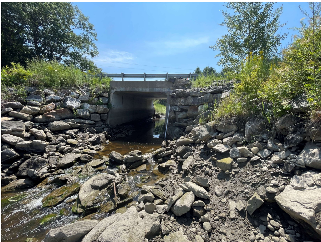
Looking upstream at existing bridge
