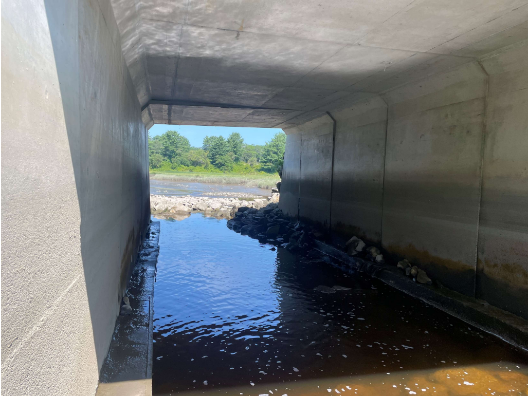
Looking Downstream through existing Bridge
