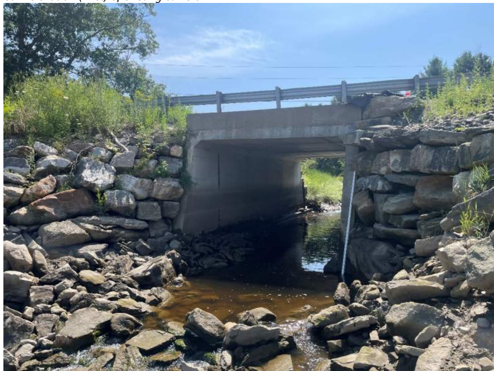
Photo 6: Downstream elevation (outlet) of existing culvert
