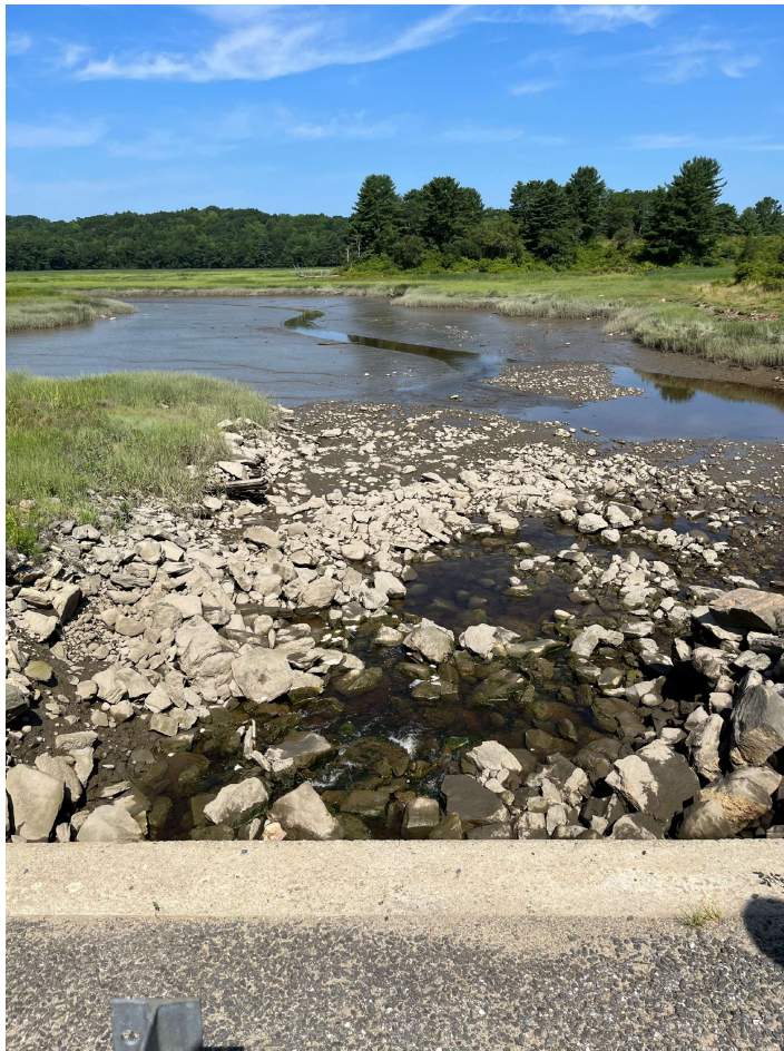
Looking Downstream from Bridge #0618
