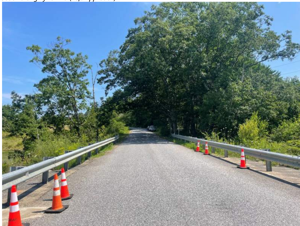
Photo 4: View North along Lynch Rd (Right Approach)
